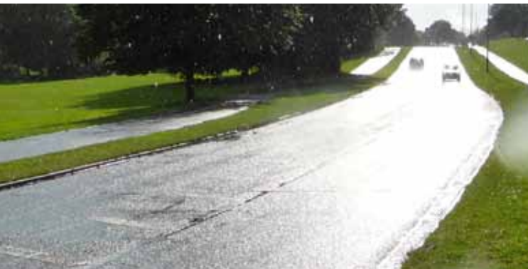
Keep in mind the angle of a rising or setting sun, as glare can pose a hazard for road users.
