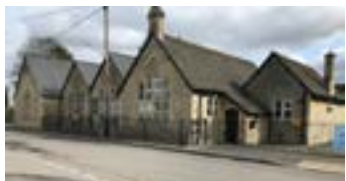
C Village Hall and Pre School
