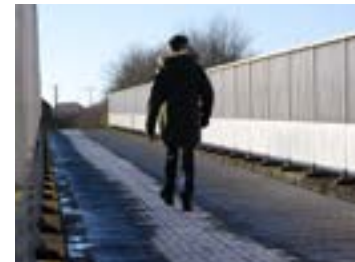
G Widhill Lane Bridleway Bridge
