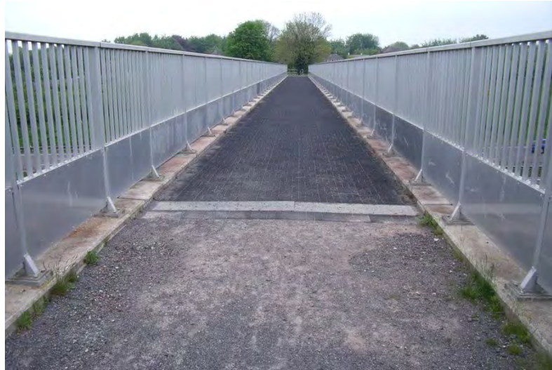
Photograph 3.1: Footbridge connection to Blunsdon
