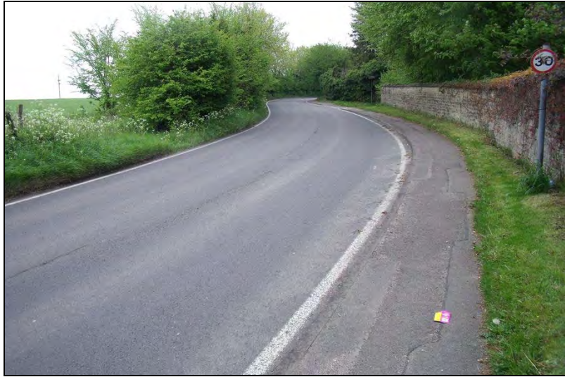
Photograph 2.(b): Tadpole Lane, looking northeast (west of the proposed development site)
