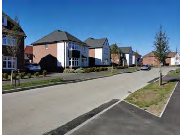
Photograph 3.5: Diamond Crescent (West), looking Northeast
