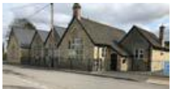
C Village Hall and Pre School
